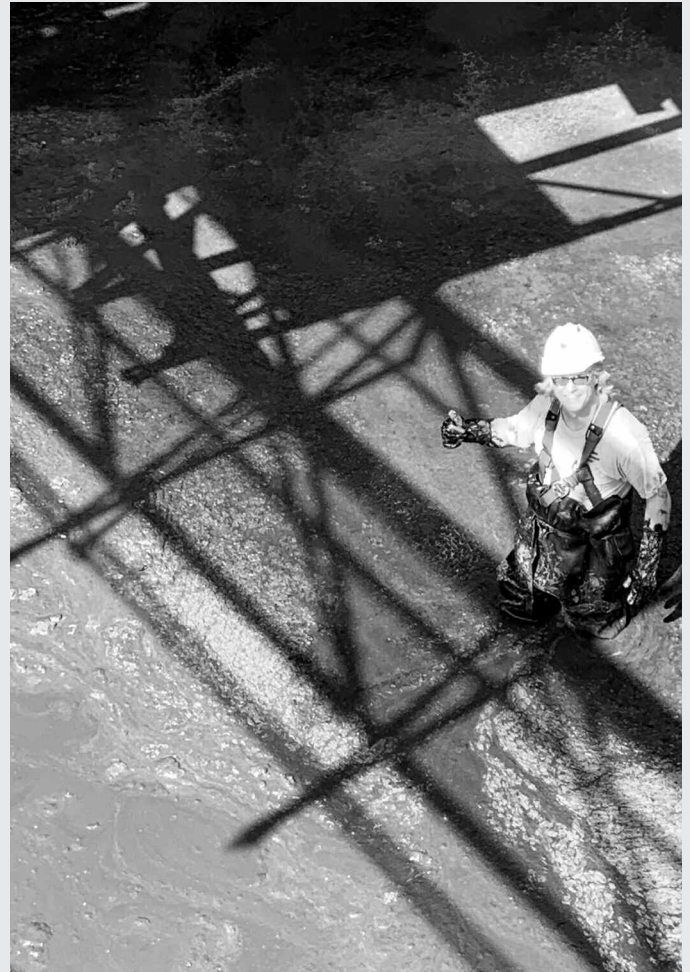
Joe Grant Working in the Primary Clarifier
